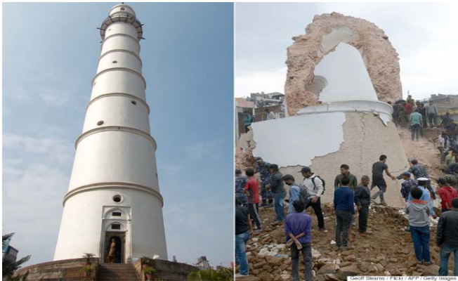
The Historic Dharahara Tower at Nepal, Before And After Collapse Due To The Devastating Seismic Effect ( It Could Have Been Avoided if the Application Of Our Research Technique Could Have Been Commercialised) occurred on 25 April 2015 at 11:56 a.m.
